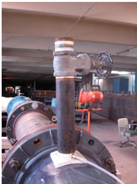
Figure 5. Air intake setup (looking upstream).
