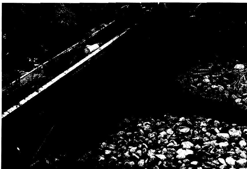
Figure 15. Solids deposition occurred both in the influent troughs and on the gravel layer.
