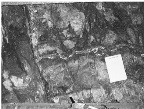
Figure 2. View of the fault zone within the Active Fault Survey Tunnel through the Mozumi fault. Field book is approximately 20 cm high. Narrow slip surface at left side of window consists of narrow clay-gouge surface; bedding is subhorizontal above the field book.
