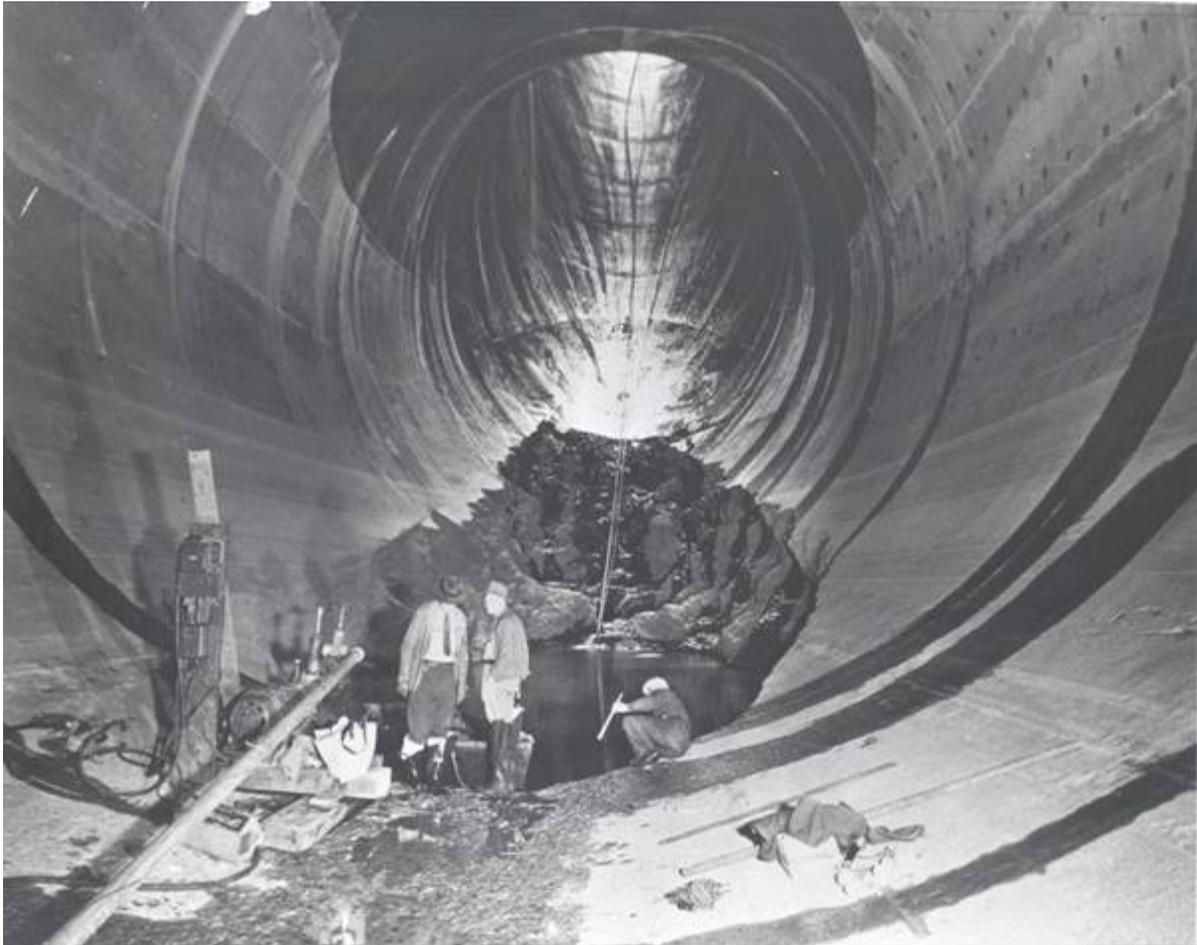
Figure 1 – Hoover Dam tunnel spillway following first substantial flows, 1941.
