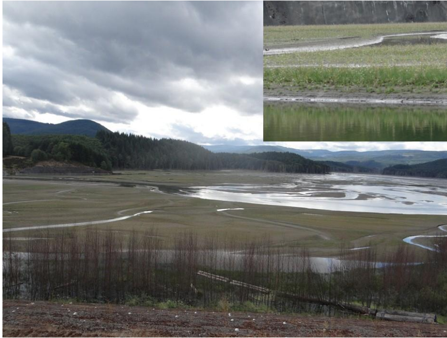
Figure 5. Conditions upstream of SRS spillway raise in summer 2013
