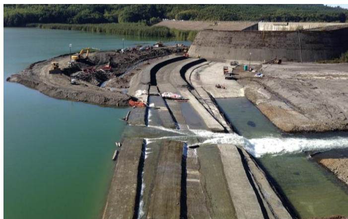
Figure 8. SRS spillway raise during construction
