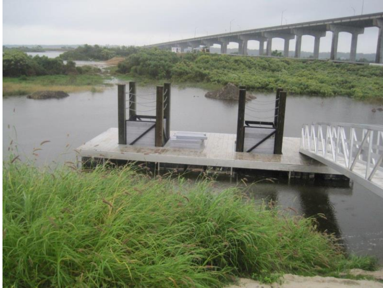
Figure 5. Bartram Island Cell F floating dock in use with composite weir boards removed and stacked on the docks deck from two sides of each box riser (Maglio et al. 2014).
