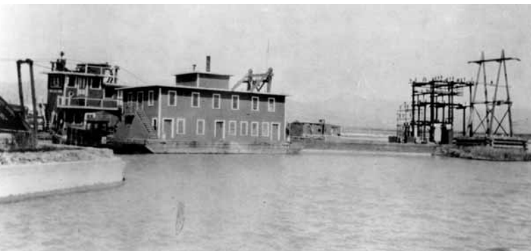
Camp Lifton on Bear Lake's north shore. Pictured here is a drag-line used to clear channel for operating Utah Power and Light's pumping station
