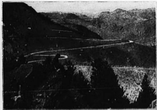
The Auto Road through Denver's Mountain Parks
