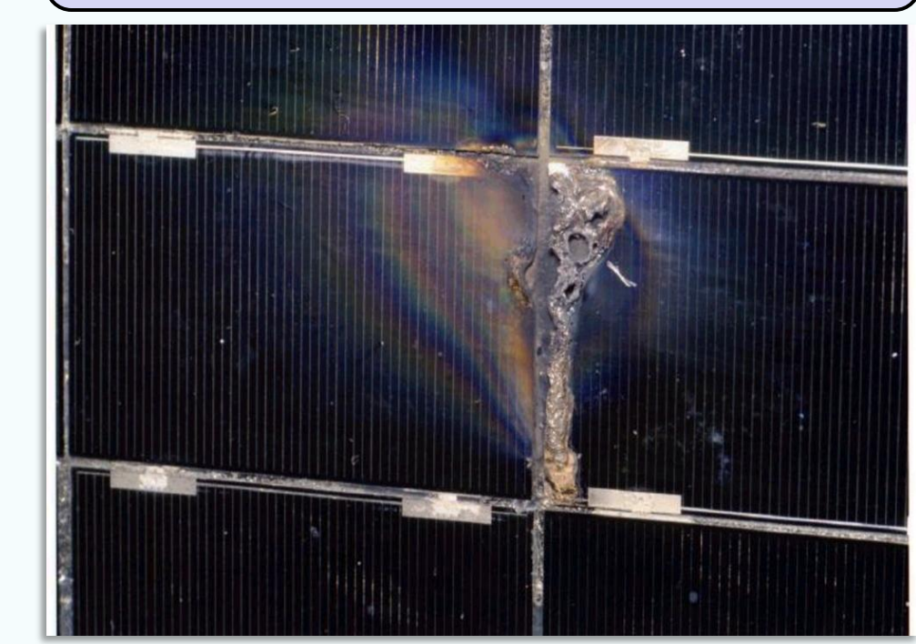
Figure 12. ESD event lead to severe damage of this solar array.
