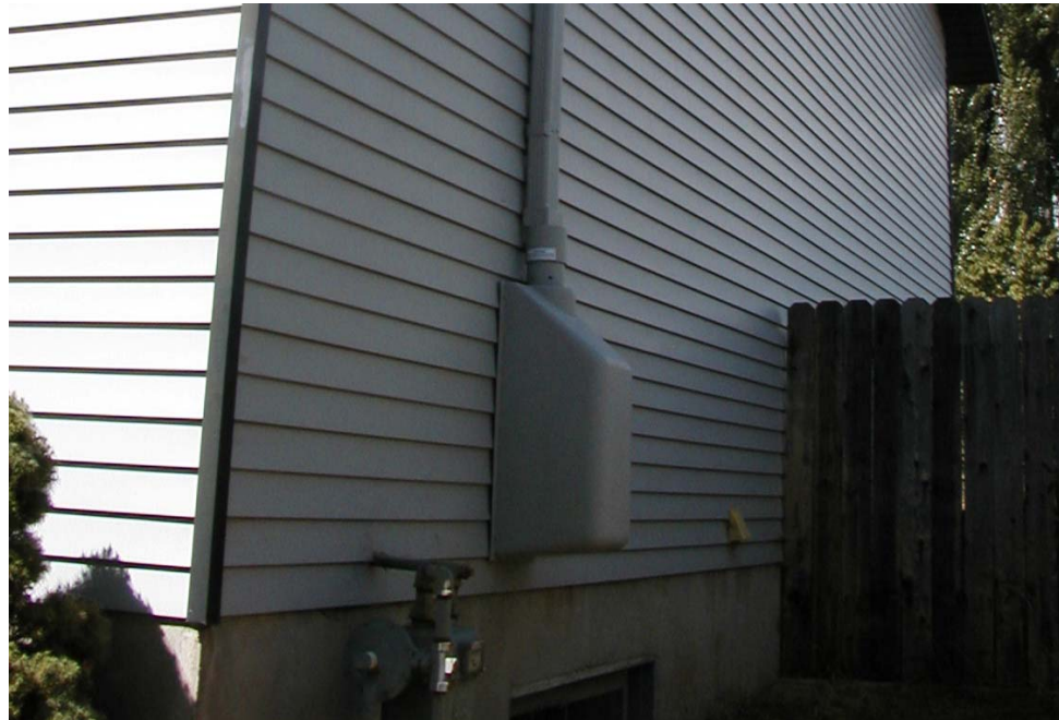
Figure 7. Exterior VRS fan installed in a residence near Hill AFB.
