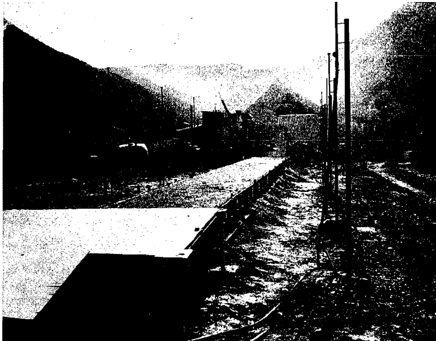
Figure 27. Concrete runoff surface during a simulation.
