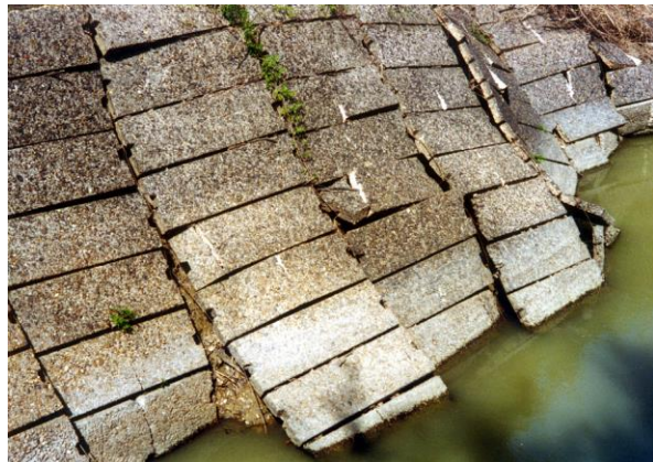
Figure 2. USACE Cable Tied Concrete
