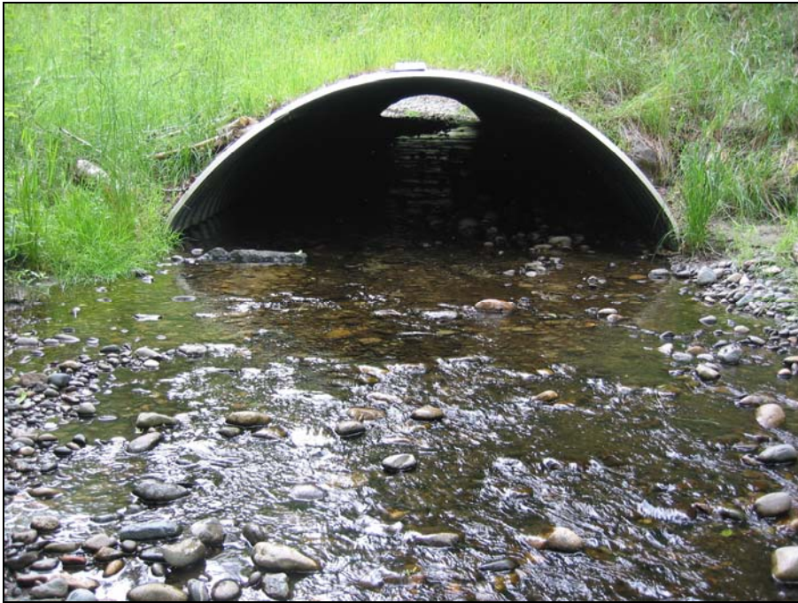
Figure 1. Example of a buried-invert culvert.
