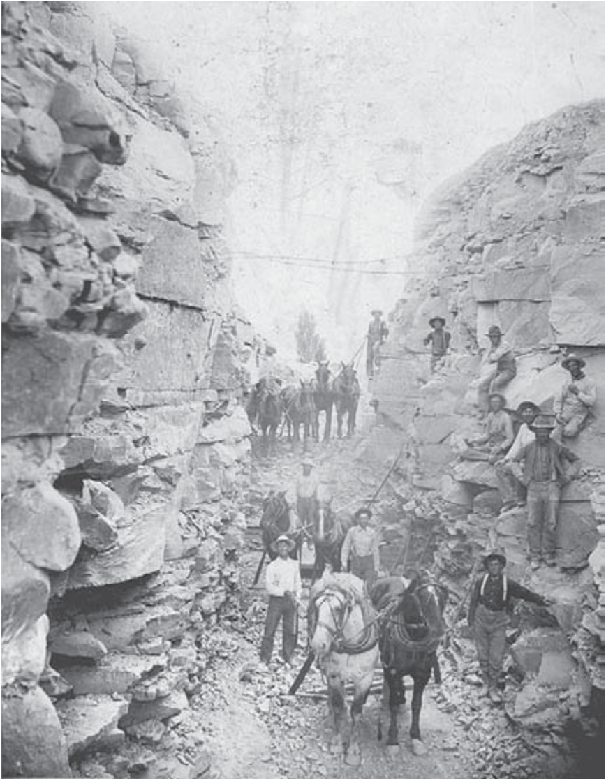
Irrigating Castle Valley meant long hours for men and teams. Here, a crew works to bring water from Muddy Creek to the area that became Moore. Courtesy of Emery County Archives.
