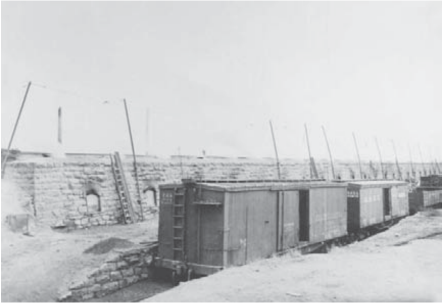
Coke ovens under construction at Sunnyside, around 1900, provided year-round work for local men, and, increasingly, immigrants from southern and eastern Europe. Courtesy of Western Mining and Railroad Museum.
