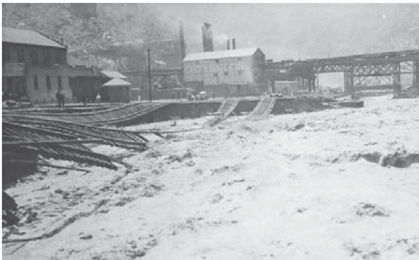
A photographer recorded the devastation at Castle Gate when the Gooseberry dam above Scofield broke in 1917. Note the warped and washed out railroad tracks at left and the splintered bridge in the background. The Castle Gate store, which remained standing, is at the far left. Courtesy of Albert Fossatt.
