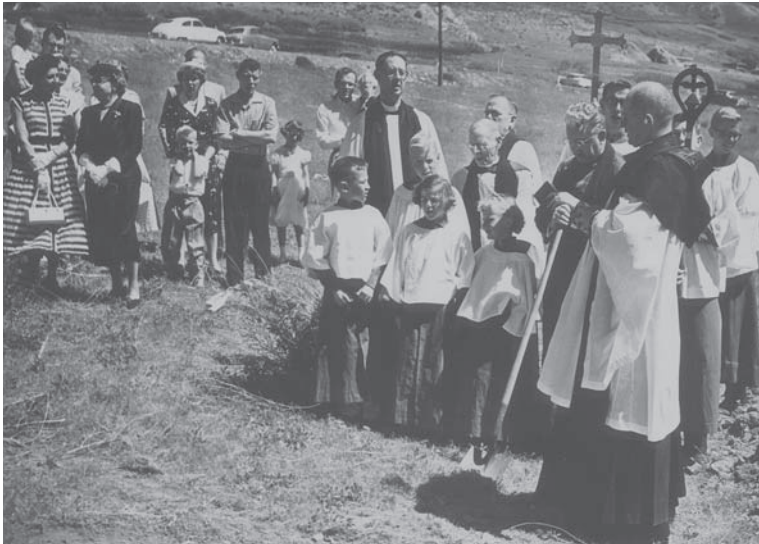
Bishop Watson (with shovel) broke ground in May 1954 for All Saints' Episcopal Church at 1710 Foothill Drive. Watson was the first Utah bishop to carry a crosier, a wooden bishop's staff, at ceremonial events. Watson's staff (visible to right) contained a Utah beehive made by the Kennecott Utah Copper Company and a lead dove from the Park City lead mines. His successor, Otis Charles, kept the crosier but removed the symbols. Diocesan Archives.
