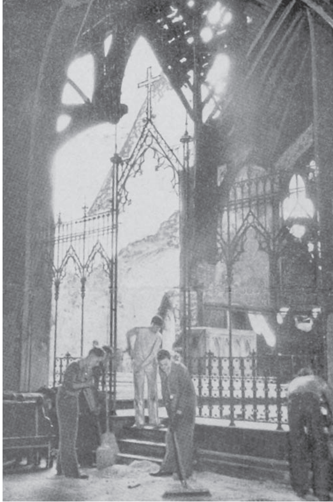
St. Mark's Cathedral sustained extensive damage in a March 31, 1935, fire caused by a defective basement furnace. Much of the sacristy was destroyed, along with several memorial windows, the organ, and altar furnishings. Cathedral membership in the early 1930s was about 600 persons; pledged income in 1932 was $6,000. Used by permission, Utah State Historical Society, all rights reserved.
