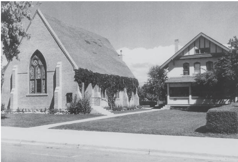
St. Paul's Church, Vernal, originally met as a congregation in 1900 in Jake Workman's Opera House, then in the Odd Fellows Hall. First services in the Gothic Revival church shown here were held on September 13, 1913. St. Paul's Lodge, next door, was completed in 1912 as a residence for single women attending schools in Vernal. It later became a hospital, then a clergy residence, and finally a parish hall. Diocesan Archives.
