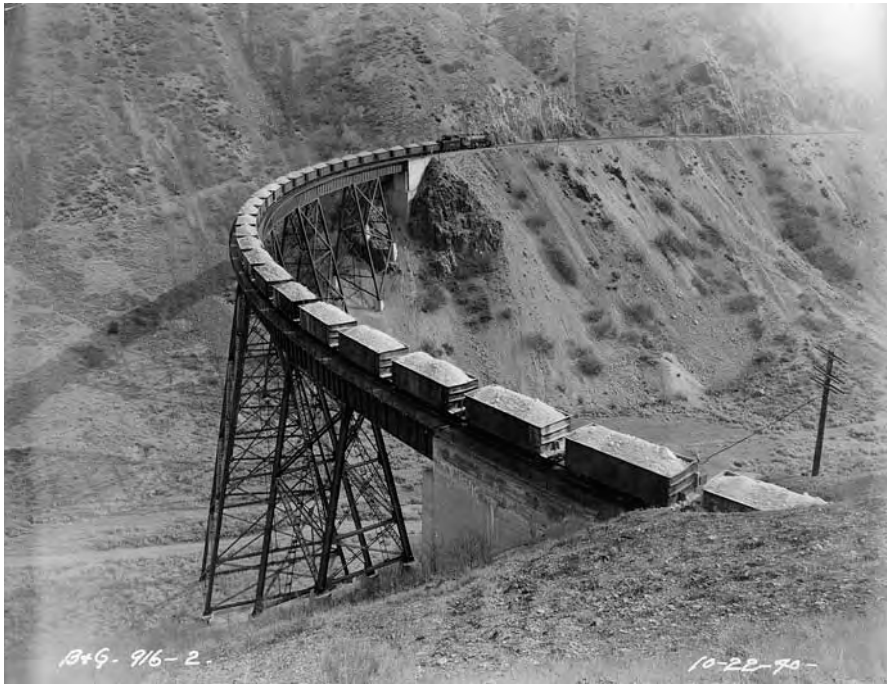
In 1940 an ore train crosses Dry Fork railroad viaduct in Bingham Canyon.
