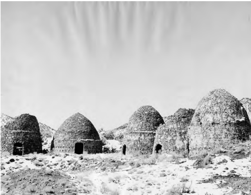
The San Francisco Mining District's distinctive beehive kilns were 20 to 24 feet in diameter and 19 to 22 feet high, with walls a foot or more thick.
