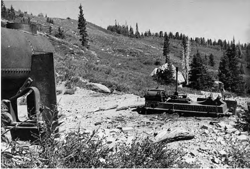
The remains of steam hoisting equipment and a boiler at Baby McKee inclined shaft in Cardiff Fork in Big Cottonwood Canyon reveal changes in mining technology. Built by Atlas Engineering Works in Indianapolis, this equipment was installed in the 1890s or early 1900s. The nearby Monte Cristo prospecting shaft (not shown), sunk during the 1917 silver boom, featured an electrically powered hoist. Photo by L. P. James (1974).
