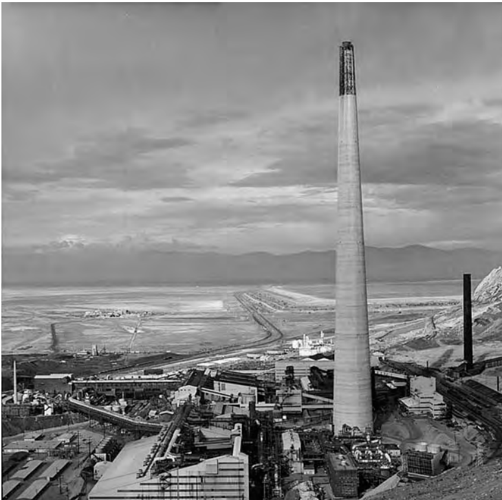
Environmental concerns and the Clean Air Act of 1970 prompted modernization of Kennecott's smelter, including this huge stack, completed in 1978, which stands 1,215 feet high.
