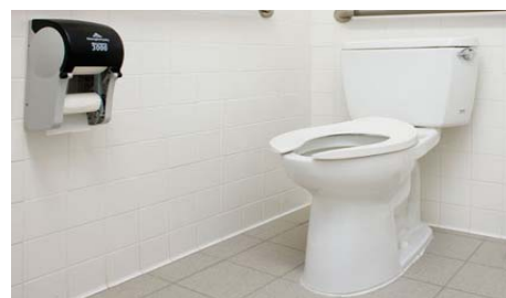
Figure 21. Low flush toilet. (LDS Church, 2010)
