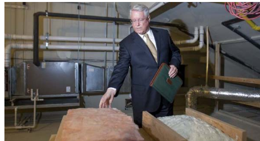
Figure 24. Efficient building insulation in meeting house. (LDS Church, 2010)
