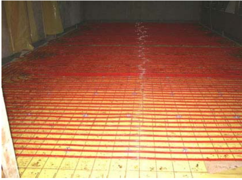
Figure 13. Construction of floor heating, Susanville CA. (LDS Church, 2010)
