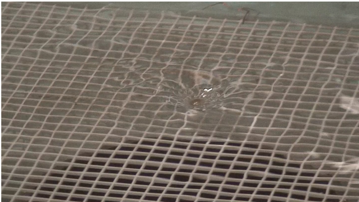
Figure 23. Debris cage with strong circulation and no air-core vortex.
