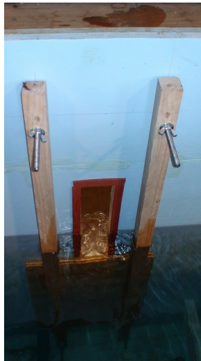
Figure 9. Overflow weir inside.
