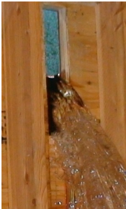
Figure 8. Overflow weir outside.
