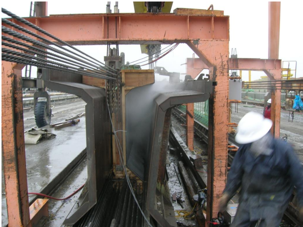
Fig. 6.3. Girders were cured in steel forms with no external steam
