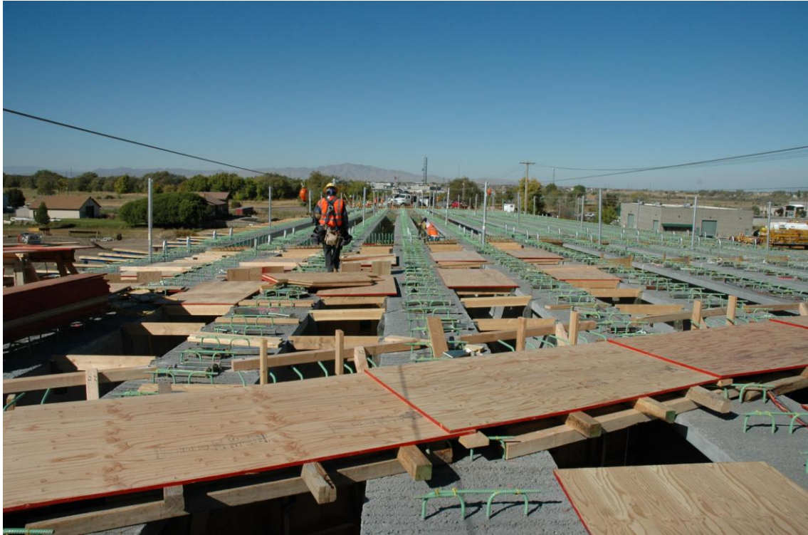
(c) Girders in place before placement of composite concrete deck
