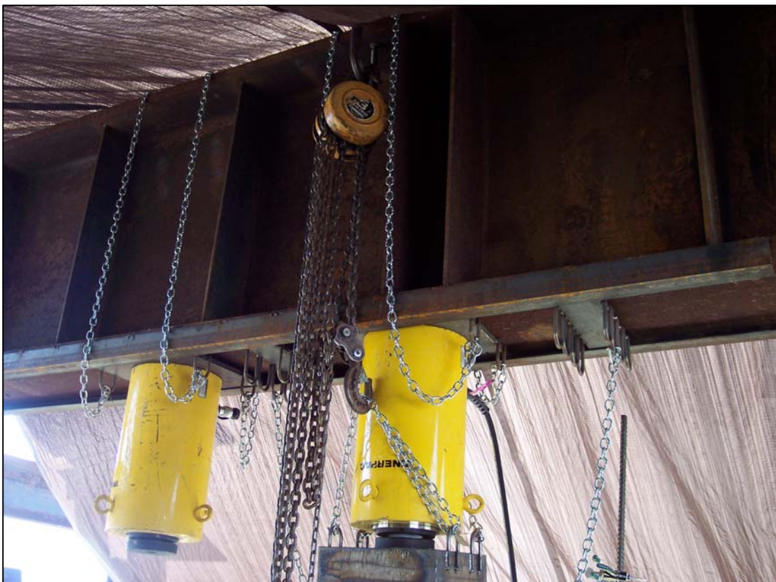
Figure 5.7. Hydraulic load cylinders.
