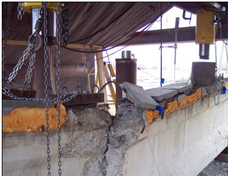
Figure 6.7. A typical flexural capacity test.
