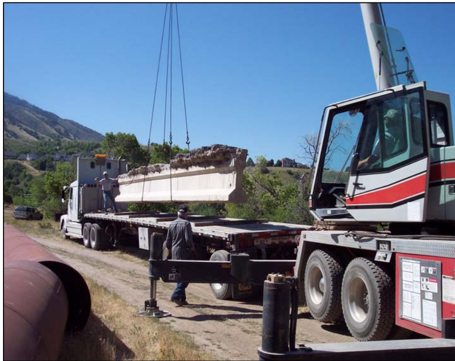
Figure 5.1. Transporting salvaged bridge girders.
