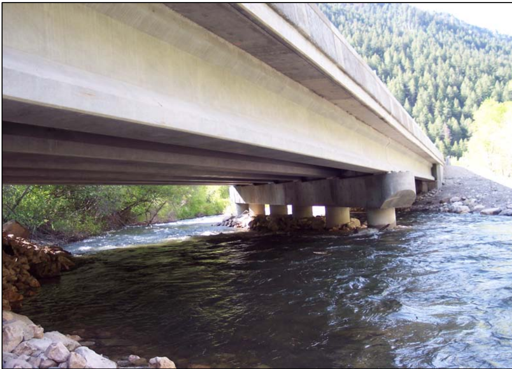
Figure 2.1. Bridge F726-3, Logan Canyon.
