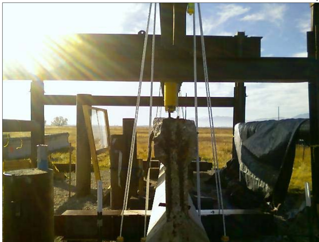
Figure 5.4. Suspending the concrete girder.
