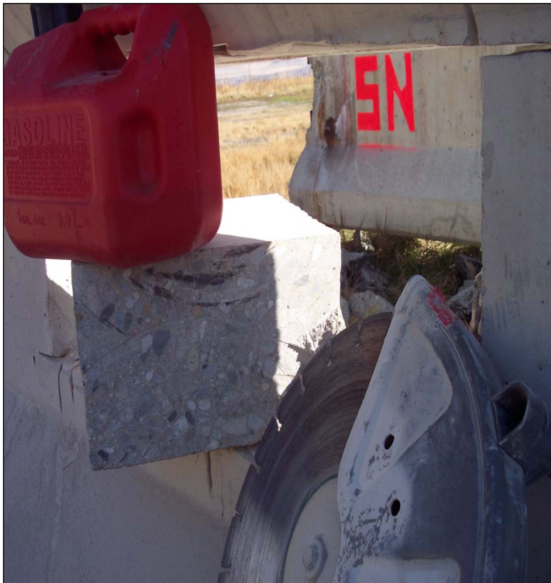
Figure 5.13. Saw-cutting a block from girder 4.
