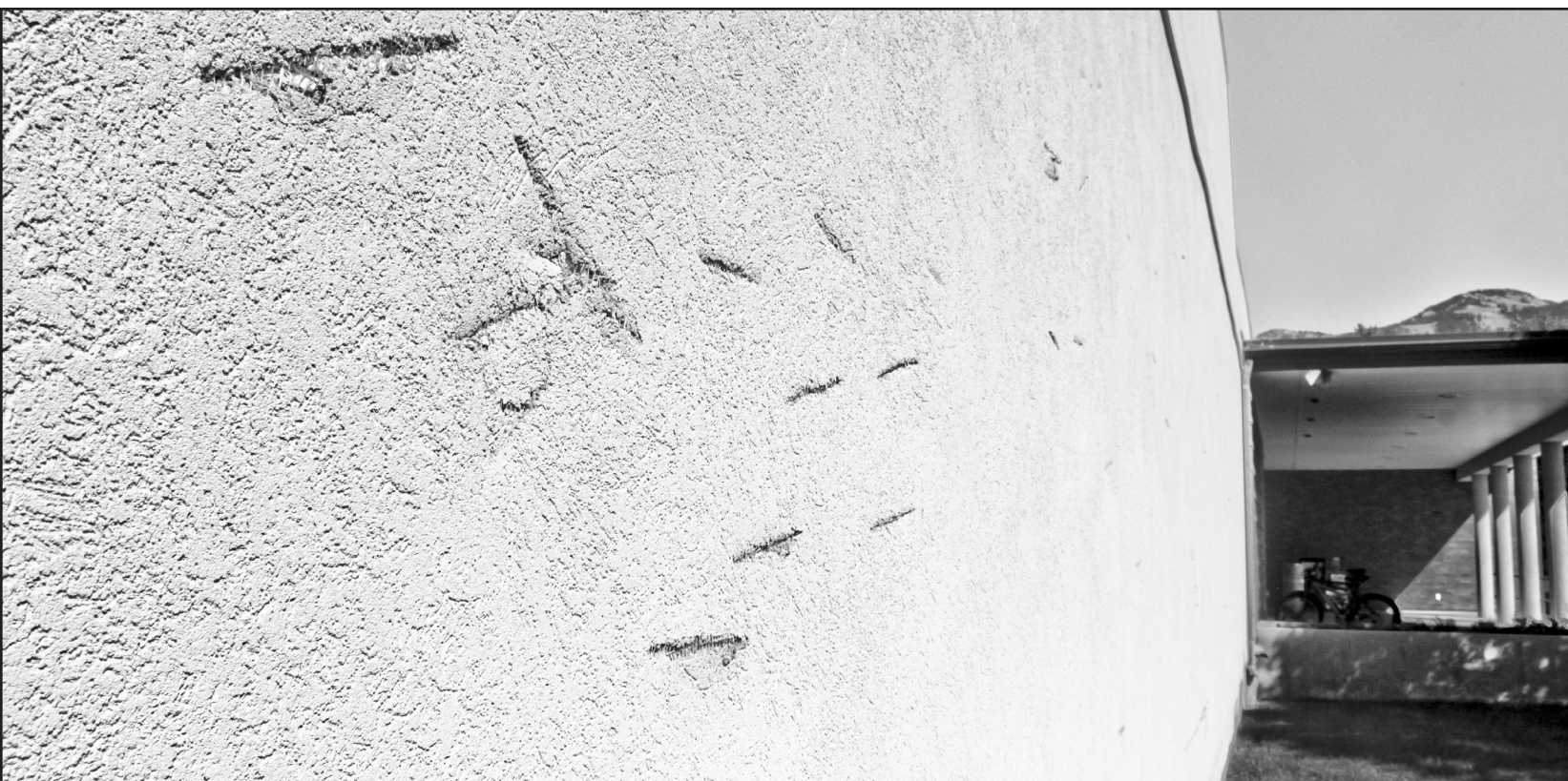
FRISBEE GOLF discs made large incisions in a wall of the Lundstrom building, which is one of the reasons it was removed from its location East of USU's campus. ALLISON OSTLER photo
