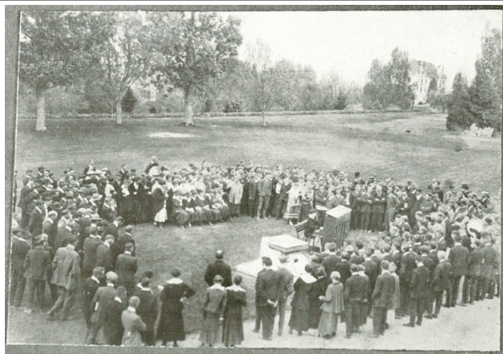
PHOTO COURTESY OF The Buzzer Photo taken from the 1917 Buzzer showing the dedication of the A block.
