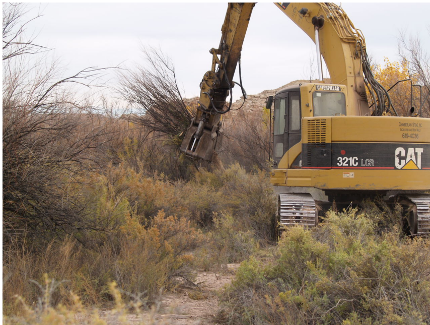
Figure 24. 321C excavator with rotary grapple attachment working to remove tamarisk at Hatt's Ranch, October 2008. This method allows individual tamarisk plants to be plucked while minimizing disturbance to surrounding native vegetation. Removal of the root ball from the soil minimizes the need for costly herbicide treatments.
