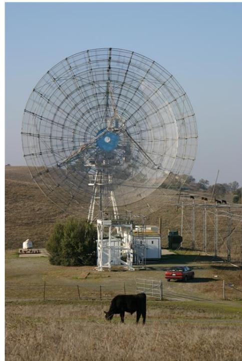
**Figure 7: SRI Earth Station 60-foot Dish Antenna**
