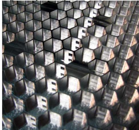
Figure 6. Detailed view of sandwich panel core illustrating wiring channel through ribs.
