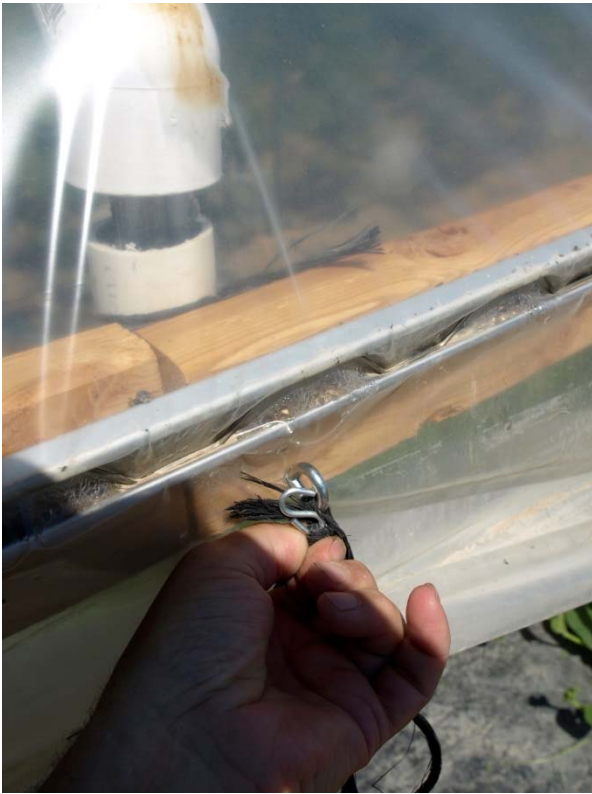
Figure 19. Lift the side curtain and use the ventilation tie to keep it up.
