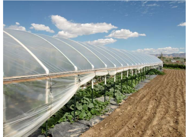
Figure 20. Lift both side curtains and open both doors for full ventilation.
