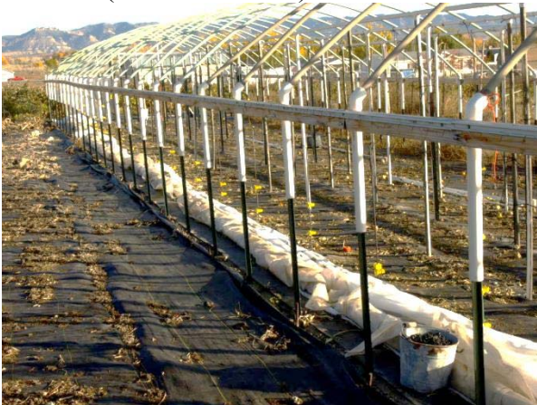
Figure 1. Note the 1.5" PVC pipes that fit over the T-posts. The T-posts are 3' apart and the high tunnel is 17.5' wide. The PVC pipe does not need to go all the way to the ground, and will be easier to remove if only 18" long.
