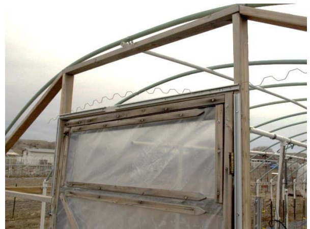
Figure 15. Wiggle wire track can be fastened to the door frame to aid in attaching the end wall plastic.
