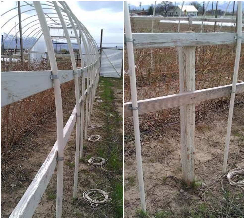
Figure 1. 2x4 side supports connected to PVC hoops and 4x4 anchor. Coils of rope attached at the base of each arch will be stretched over the tunnel to further tension the plastic.
