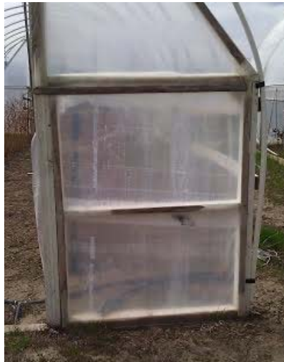
Diagram 3. Main door, one side only. Two of the above doors should be constructed and hung so they will open as double doors
