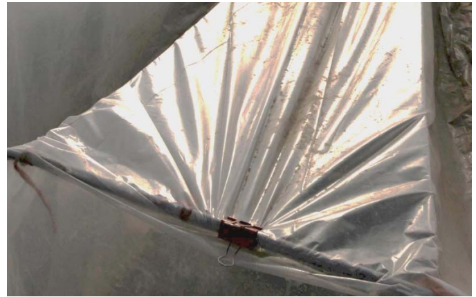
Image 7. Binder clip securing plastic to conduit frame.
