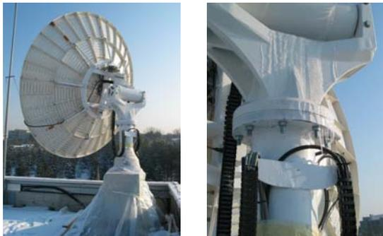
**Figure 14- Ground station dish:** Due to freezing snow, the joints of ground station dish have been frozen many times
