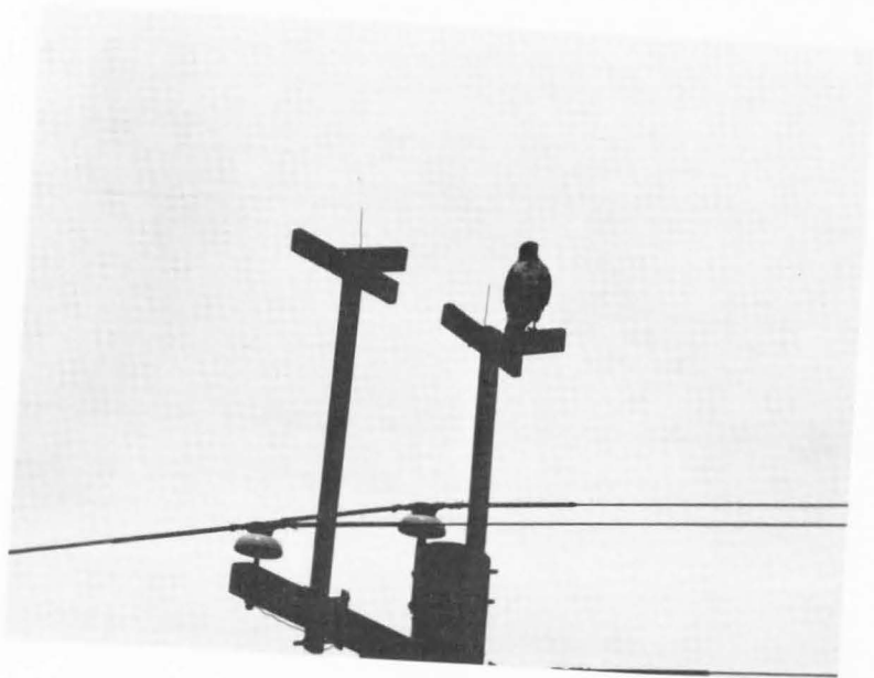
Figure 7. Electric utility pole with perches constructed by the USAF, being used by a red-tailed hawk. Note insulators mounted above cross-bars. (Photograph taken on Hill Air Force Range, western Utah).
