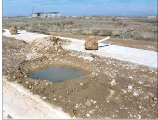
Drainage problem in a tree planting hole. The problem could be solved by the installation of a vertical drain before planting.
