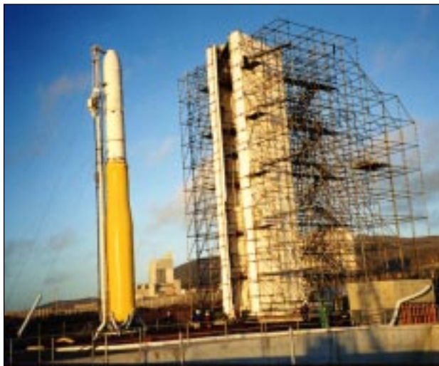
Figure 16 - Minotaur with Thermal Blanket and Retracted Scaffold
