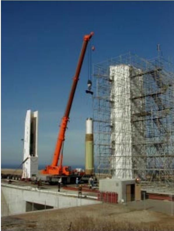
**Figure 14 - Lower Stack Assembly Emplacement**
