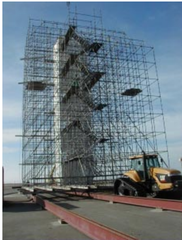
Figure 15 - Environmental Protection and Access System with Tug
