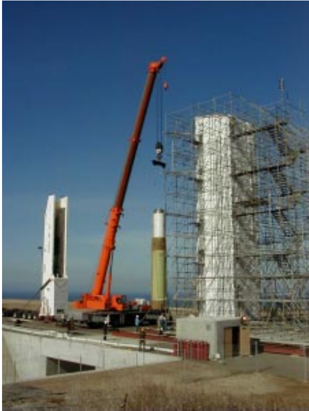
Figure 14 - Lower Stack Assembly Emplacement
