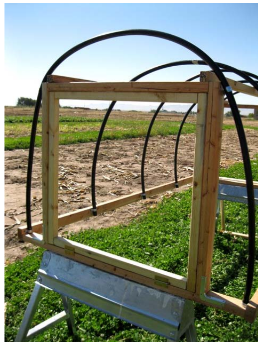
Figure 5. Tunnel frame assembled before installation of vents and plastic.
