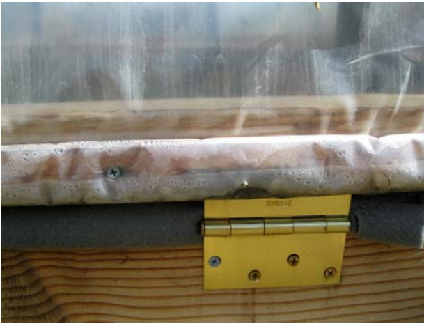
Figure 6. Plastic rolled over lath and screwed onto board I/J.
