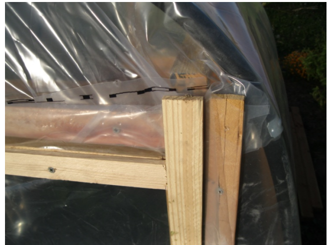
Figure 8. Closed vent. Note how the lath and plastic are situated to cover the gap between the vent frame and vent.
