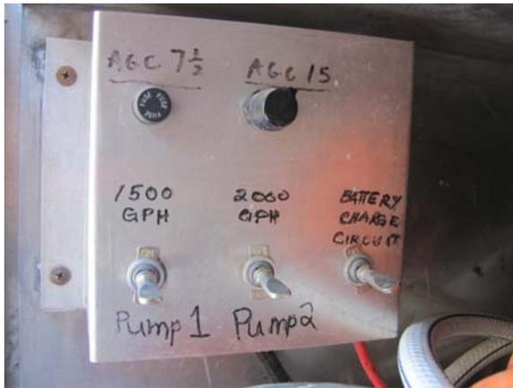
Picture G: Pump switch/fuses
