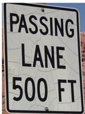
D. Cracking Damage
