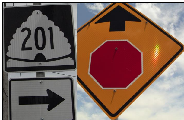
FIGURE 3.5 Improperly oriented Type III HIP sheeting
