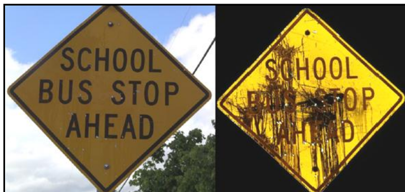
FIGURE 3.7 Illegible traffic sign caused by vandalism damage
