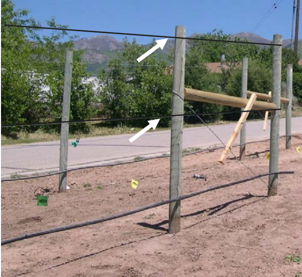
Figure 1. A 2-wire vertical trellis suitable for the Kniffen training system, with wires (white arrows) at 36 and 60 inches above ground level. This view shows the end braces with cross bar and diagonal tensioned wire. A drip irrigation line is suspended approximately 1 foot above the ground.
