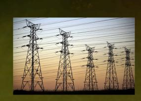
Electric power industry - power companies transmit alternating current to their customers via long transmission lines. Direct currents induced in these lines from geomagnetic storms are harmful to electrical transmission equipment. In 1989 a geomagnetic storm trigged the collapse of the Hydro-Quebec power grid, leaving 6 million Canadians without power for 9 hours.
