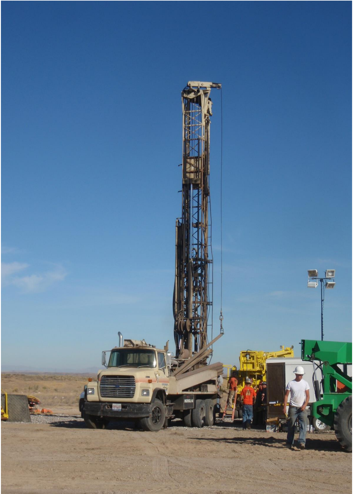
Figure 5. Eaton Drilling & Pump Service setting surface conductor casing.
