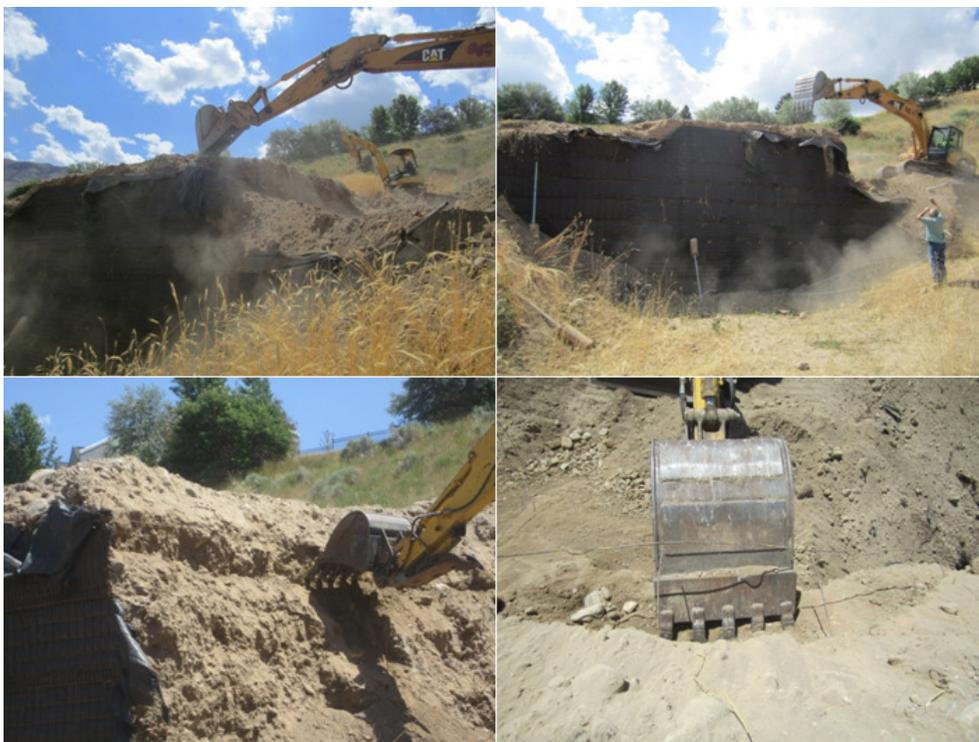
**Fig. 3.24.** Exhuming of USU Wall
