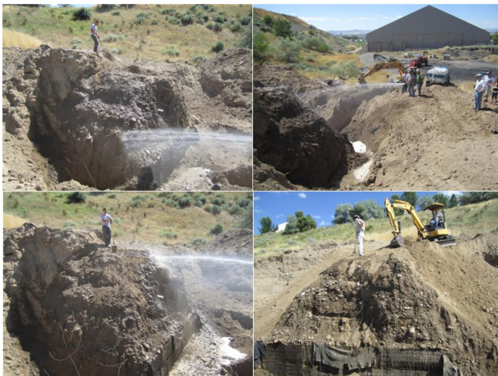
**Fig. 3.25.** Exhuming USU Wall using a water hose
