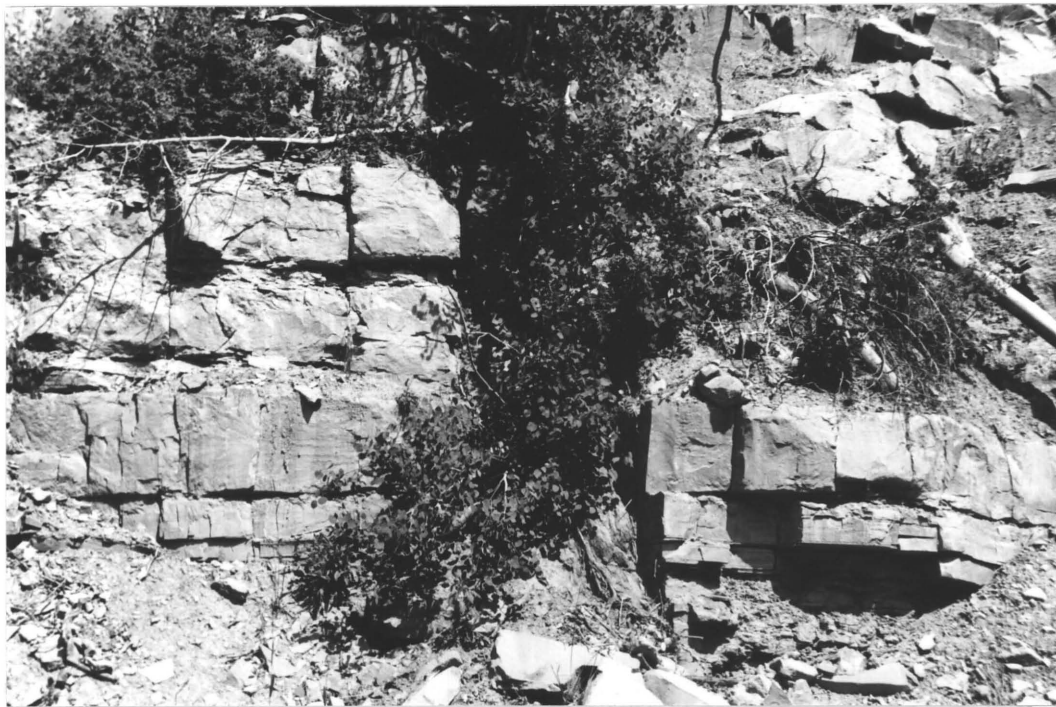
Figure 4. Weathered dike exposed in road cut along northern side of Boardinghouse Canyon, west of Clear Creek, Utah; view west. Dike is along a joint. Dike is also illustrated in Figure 2.
