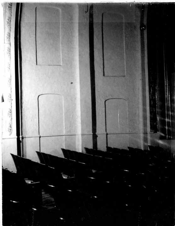
Figure 17. Opening that used to house the old box seats. (These were closed off during a later remodeling.)
