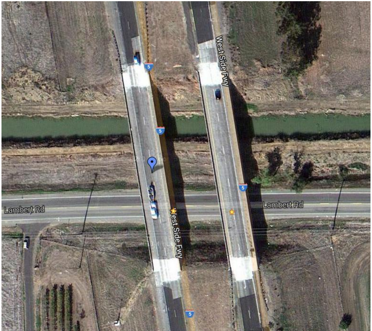
Figure 2. Aerial view of the 24-0287L Bridge (blue marker). North up.
