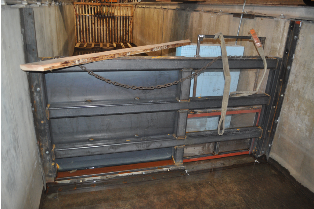
Figure 9. Model A prototype structure installed in 8-foot flume (looking upstream).
