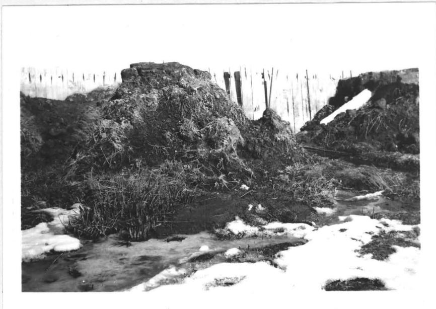
Figure 5. Break in dike 120 yards east of Teal Spillway. Basic cause of break was non-rock fill on old stream channel; secondarily by muskrats.
