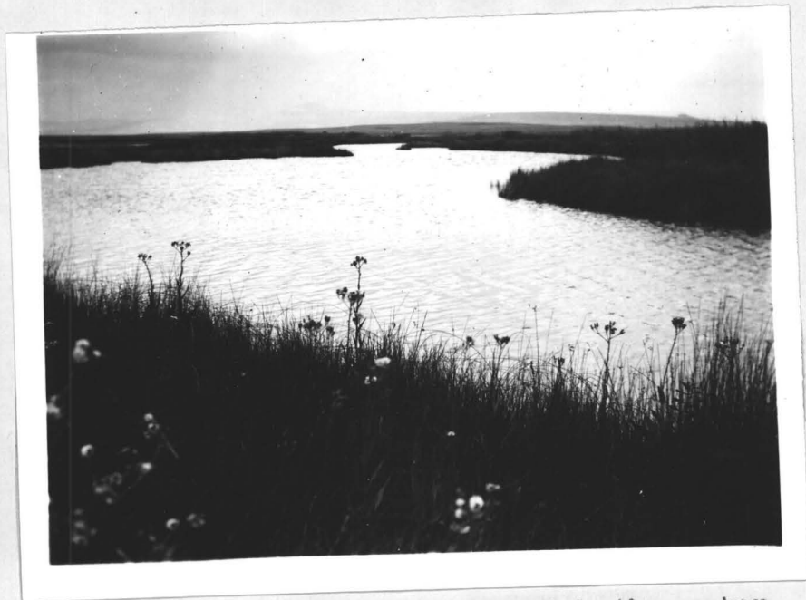
Figure 3. Baker's Spring run with the water turned on at Baker's Spillway to water some far knolls.
