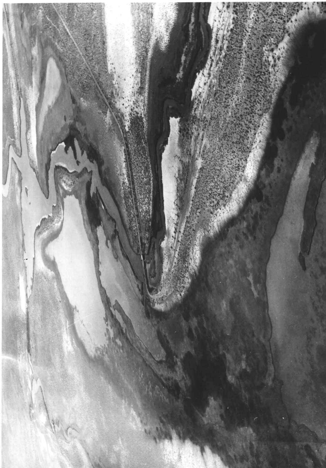
Figure 29. Aerial photograph of Baker's Spring showing the spillway and interconnecting canals.
