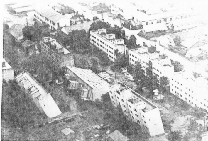
Figure 3-8. Foundation failures in Niigata, Japan (1964) (after Seed, 1975a).
