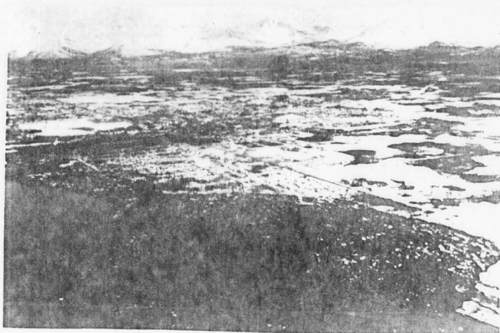
Figure 3-9. Turnagain Heights landslide, Anchorage, Alaska (1964) (after Seed, 1975a).
