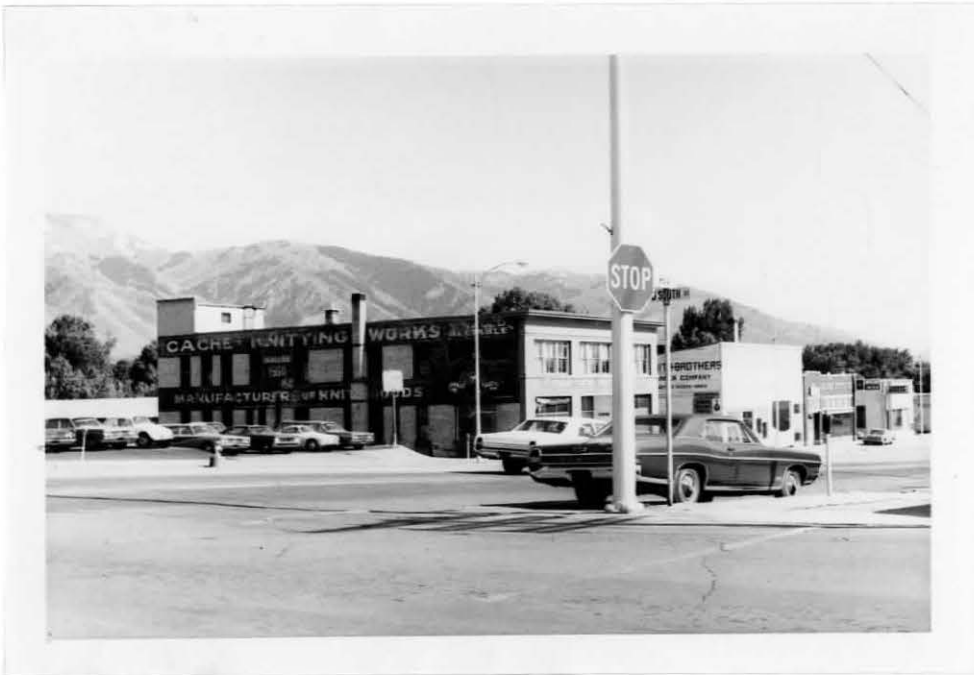
Figure 30. Warehouse building in the central business district.
