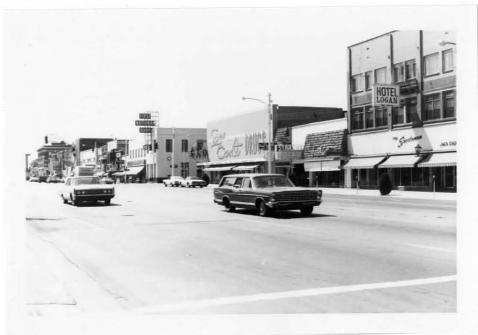
Figure 26. Main Street traffic facing south.
