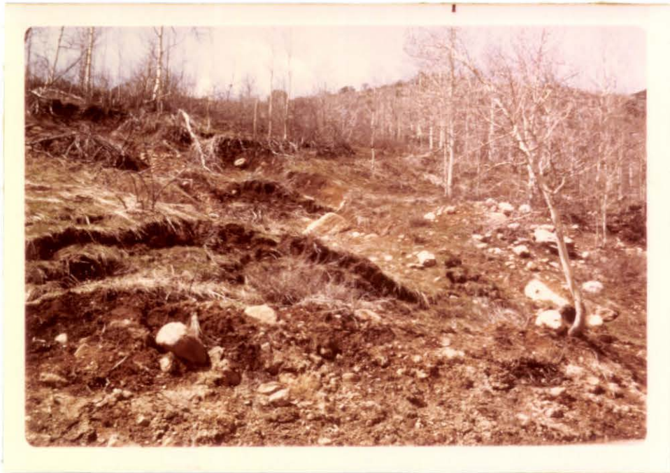
Photograph 2. Sliding failure of unstable soil
