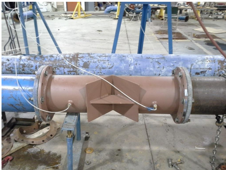
Fig. 10. Wedge flow meter installation.
