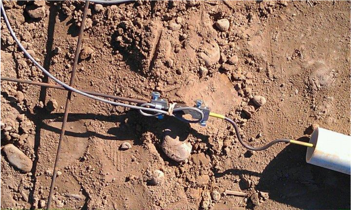
Figure 3.6 Installed In-Line Load Sensor
