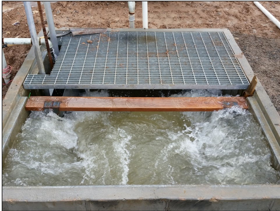
Figure 20. Prototype splitter box before vertical plate was installed.
